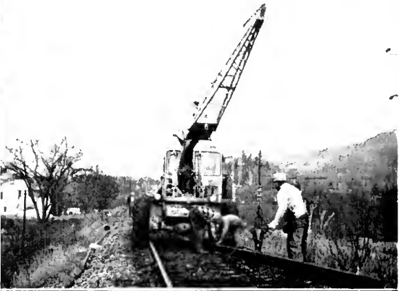
LAYING STANDARD RAIL
